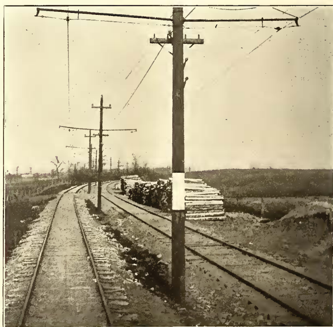
OVERHEAD WORK AT DOUBLE-TRACK CURVE, C., L. & S.
